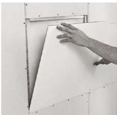
**3** Insert the speaker into the prepared recess. Make sure that there is no strain between underlying insulation and panel (no compression). The speaker should be easily insertable into the opening.
