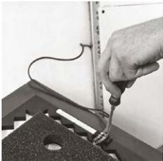
**2** The enclosed cable lugs have to be properly crimped to the connector cable. Then connect the cables following the colour coding / markings, for example, marking to plus (red). This order has to be maintained building and amplifierwise.
