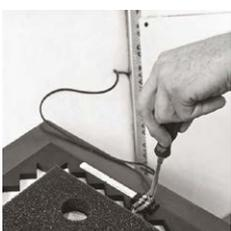
**6** The enclosed cable lugs have to be properly crimped to the connector cable. Then connect the cables to the connector terminal paying attention to the polarity.
