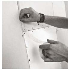
**6** As it is obligatory with single-ply plasterboard constructions, the joints between plasterboard and speaker have to be always filled with a crack bridge. The same filling material that is used against cracks in other joints can be also applied here.
