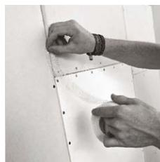
**10** The joints between wall/ceiling and the speaker panel have to be filled with a crack bridge.
