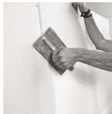
**8** Cerasonar speaker panels are out-fitted with a primer and have to be spackled all-over with the surrounding surface. Thus, Q3 and Q4 wall / ceiling qualities are easily possible.
