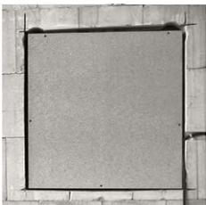
**2** The frame is ideally mounted flush to the finished wall surface. Therefore the wall plaster should have been applied to the masonry already, so that the speaker only has to be fine spackled flush to the wall surface using a fine or structured filler. The connector cable has to be installed into the frame before.
