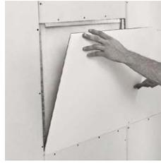
**7** Insert the speaker into the prepared recess. Make sure that there is no strain between underlying insulation and panel.
